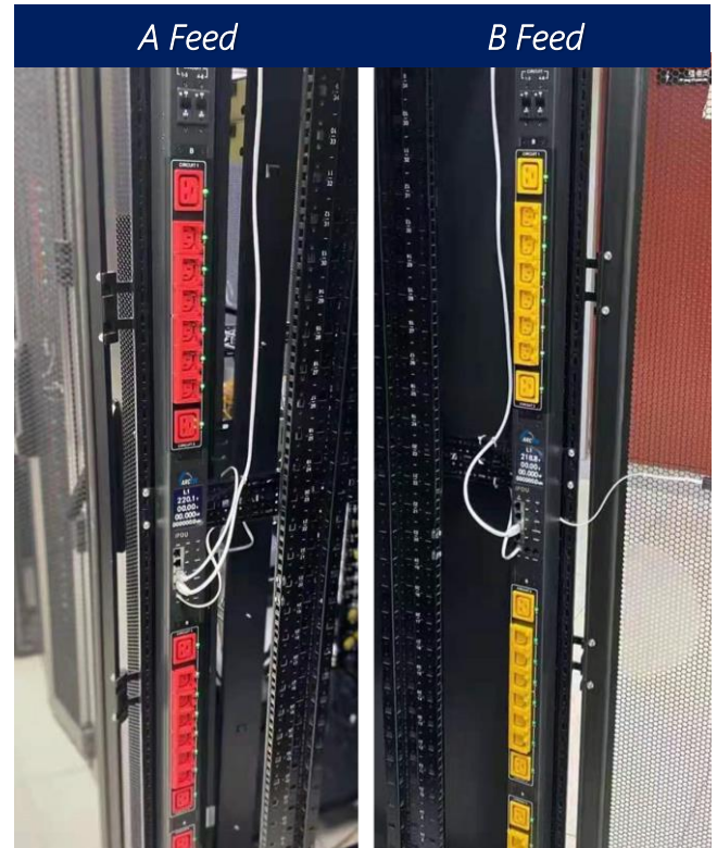
Colored Outlet Modules, by A & B Feeds
